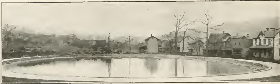
The pool as it looks today completed. The floor of the pool gradually slopes toward the center where it is deep enough for diving.
